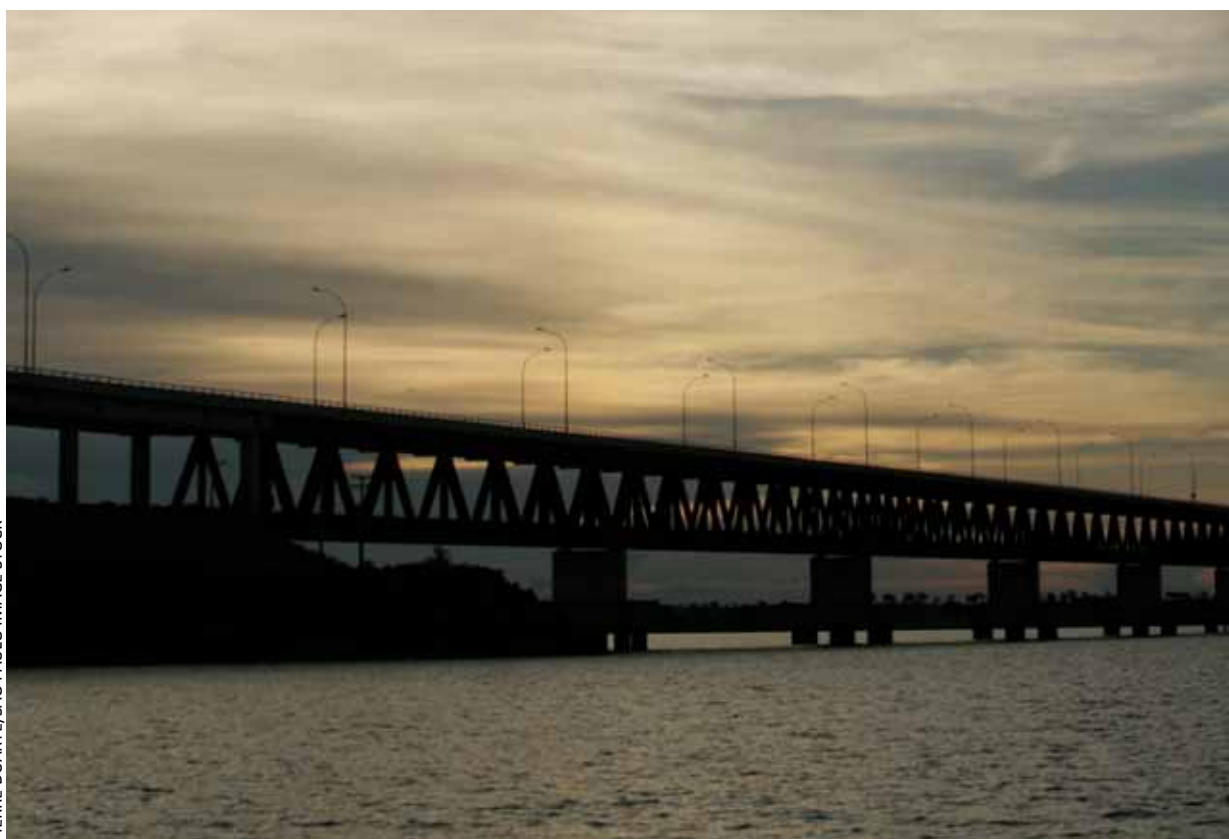
Road-rail bridge in Rubinéia, SP. 2600 meters long, 10 meters high and 15 meters wide, it is the world's largest road-rail bridge of its kind.
