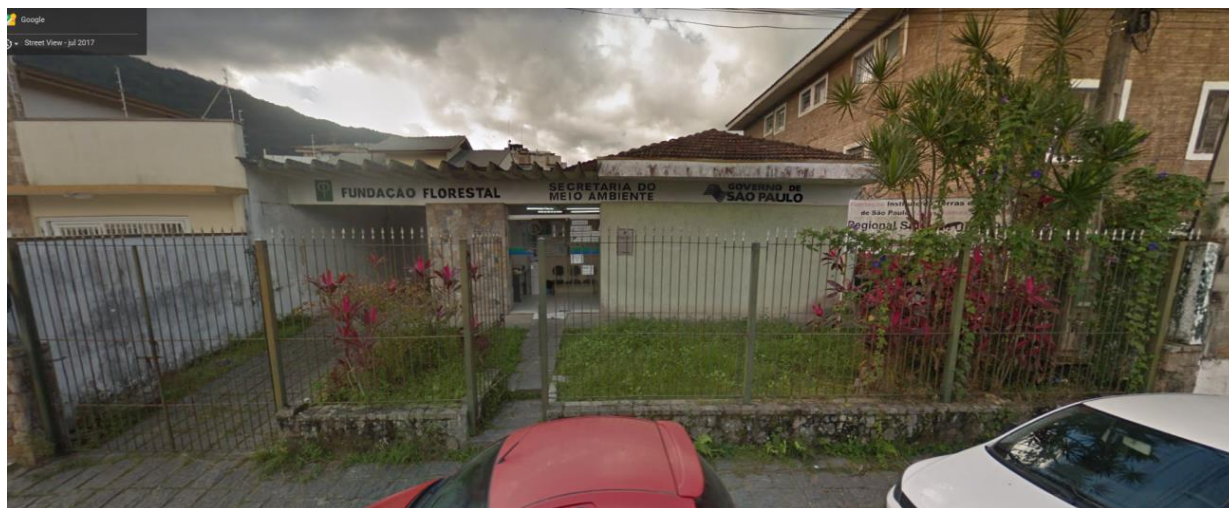
Figura 3 – Fachada frontal (Google Street View).
