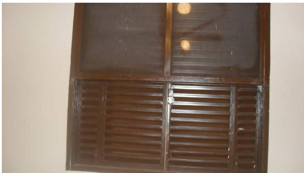
Foto 27 – As guilhotinas emperram, necessitam de ajustes
